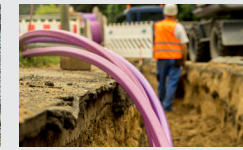
200 psi: Cable blowing and drilling
